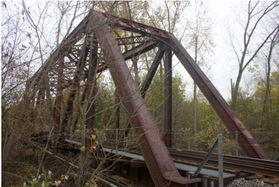
View of Caledonia's southernmost (Big Four) railway bridge, facing Northwest. October 2022.
